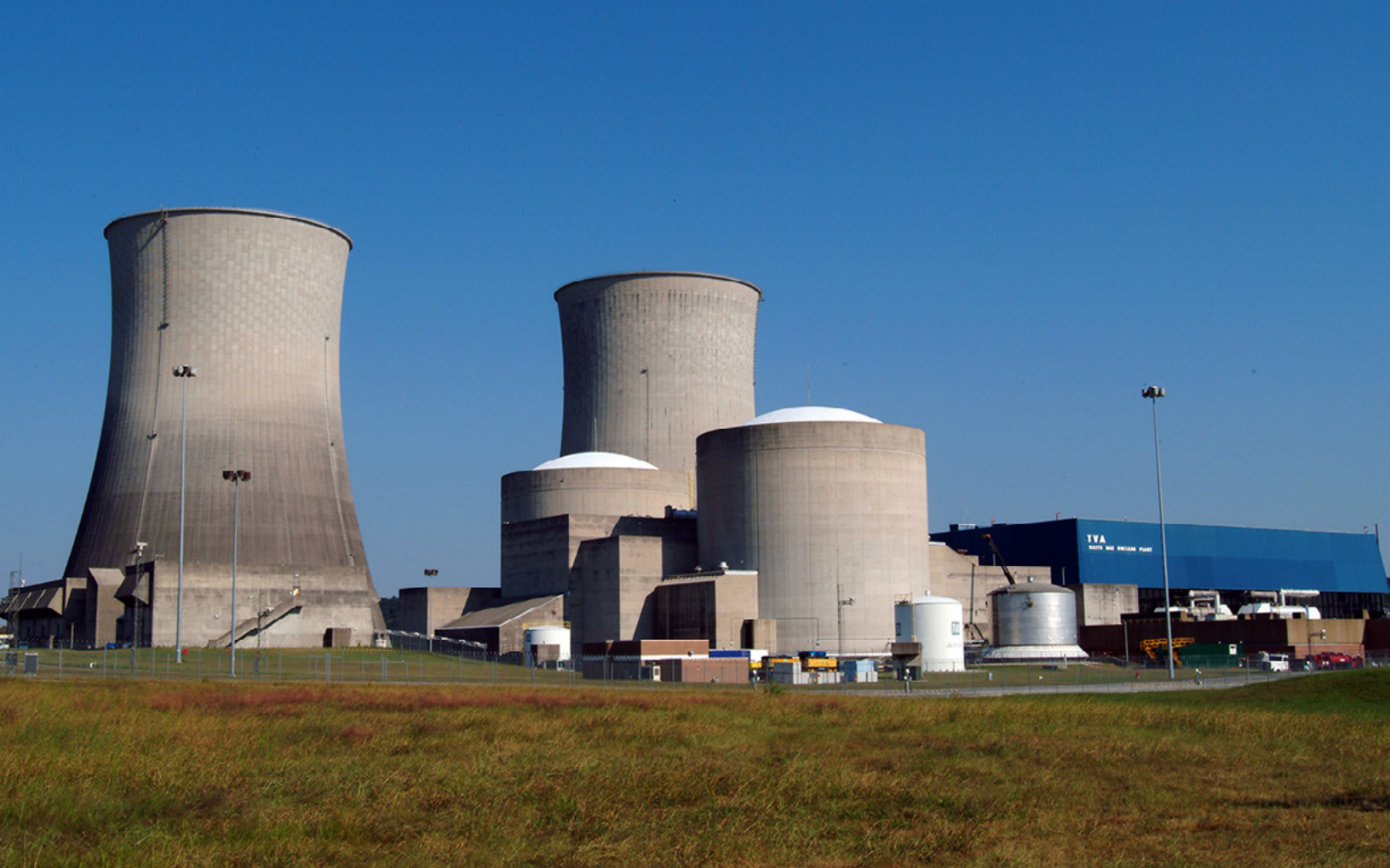
Unit 1 of the Watts Bar Power Plant, operated by the Tennessee Valley Authority, is the only reactor producing tritium for U.S. nuclear weapons. A second reactor at the site is expected to begin supplementing tritium production in 2020. (Photo: Tennessee Valley Authority)
