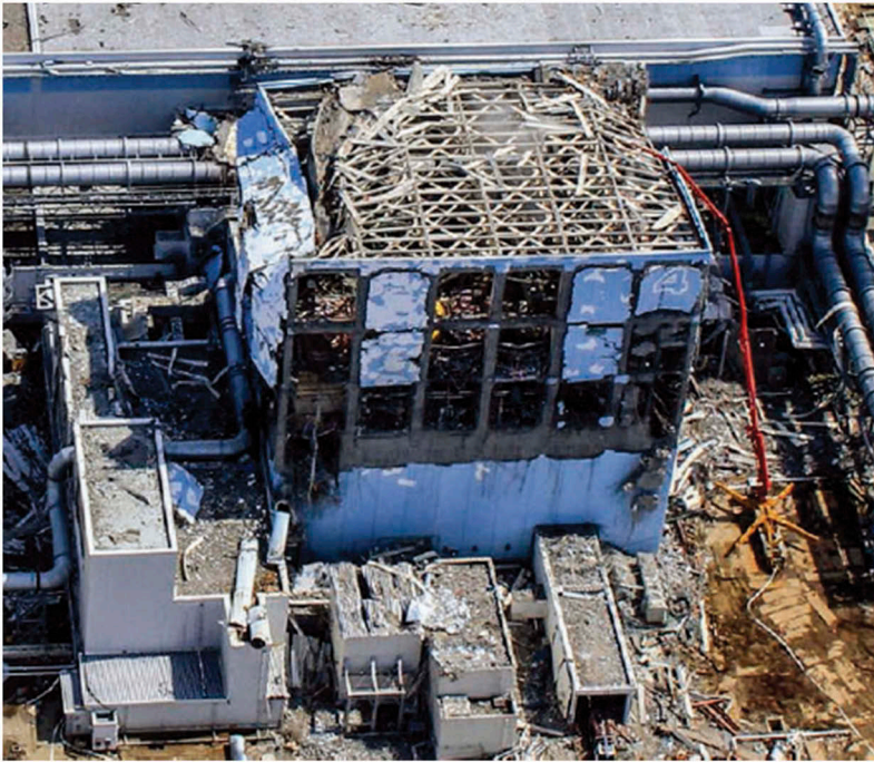
Figure 2. Fukushima Daiichi Reactor Building 4 after the hydrogen explosion on 15 March 2011. On the right is the “giraffe,” a cement pump whose boom was used to deliver water to the pool through a hole in the roof (TEPCO).
