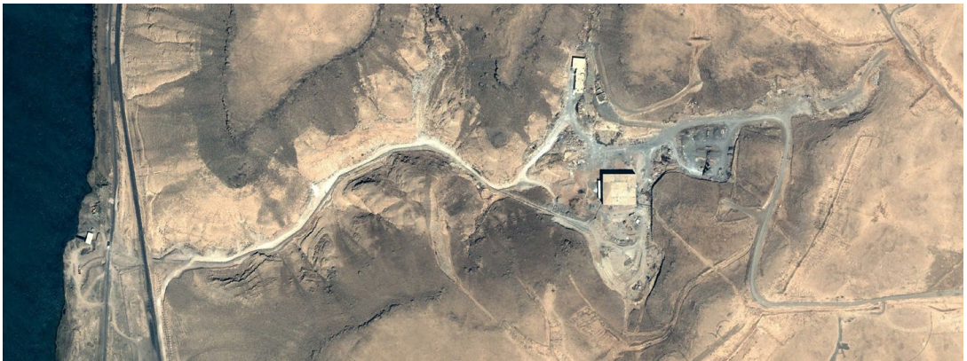
The Al Kibar site (35.708 N, 39.833 E) in Syria in August 2007, shortly before it was destroyed by Israeli aircraft. The construction of an undeclared plutonium production reactor had apparently been underway, 40 possibly with foreign assistance. Credit: Google Earth.
