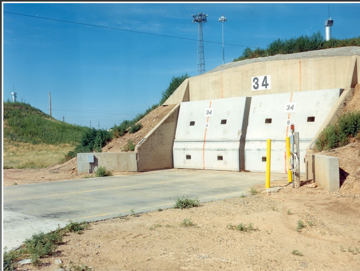
Entrance to Storage Magazine at Pantex, Zone 4 Uses 40-ton concrete blocks to prevent unauthorized access Credit: U.S. DOE
