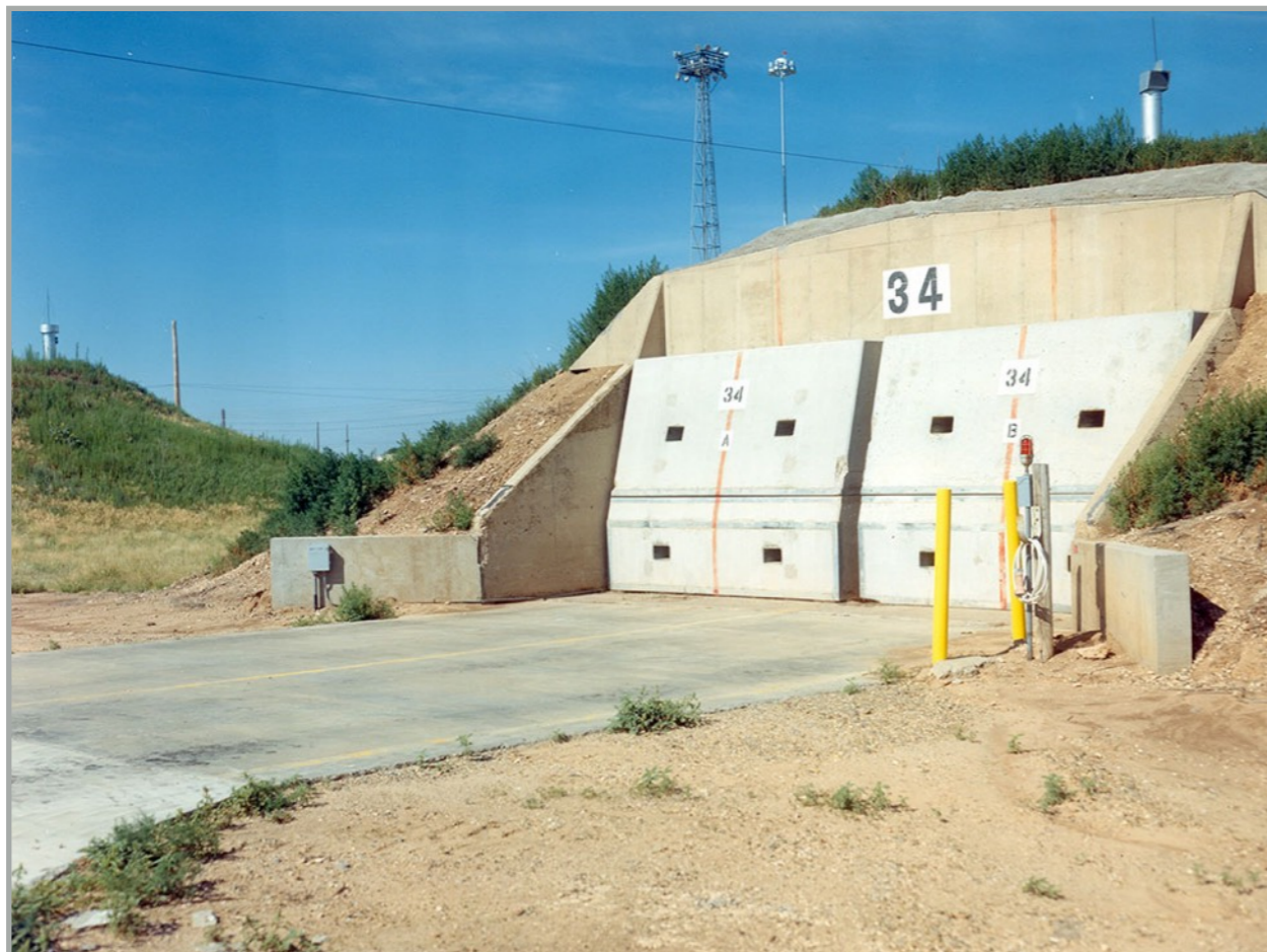
Entrance to Storage Magazine at Pantex, Zone 4 Uses massive concrete blocks to prevent unauthorized access Credit: U.S. DOE
