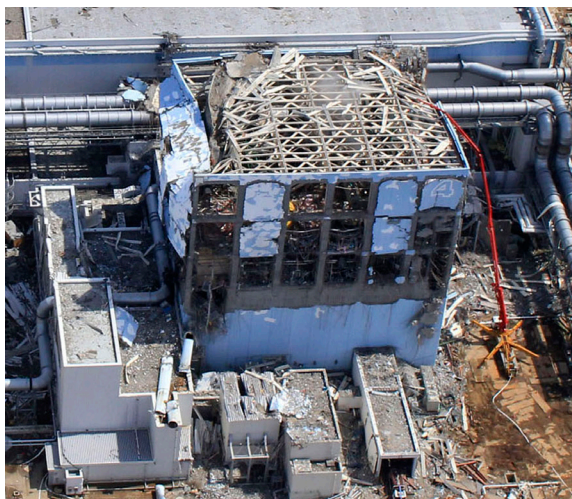
Unit 4 at the Fukushima Daiichi nuclear power plant, damaged by an explosion on 15 March 2011.
