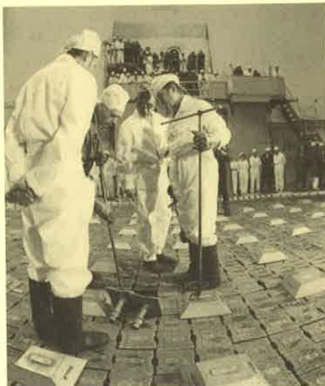
Fig. 7 Top of one of the shut-down Krasnoyarsk-26 reactors. Each square covers one channel. The raised covers indicate the locations of control rods. The two pipe tops show the diameter of the fuel channels. 7
